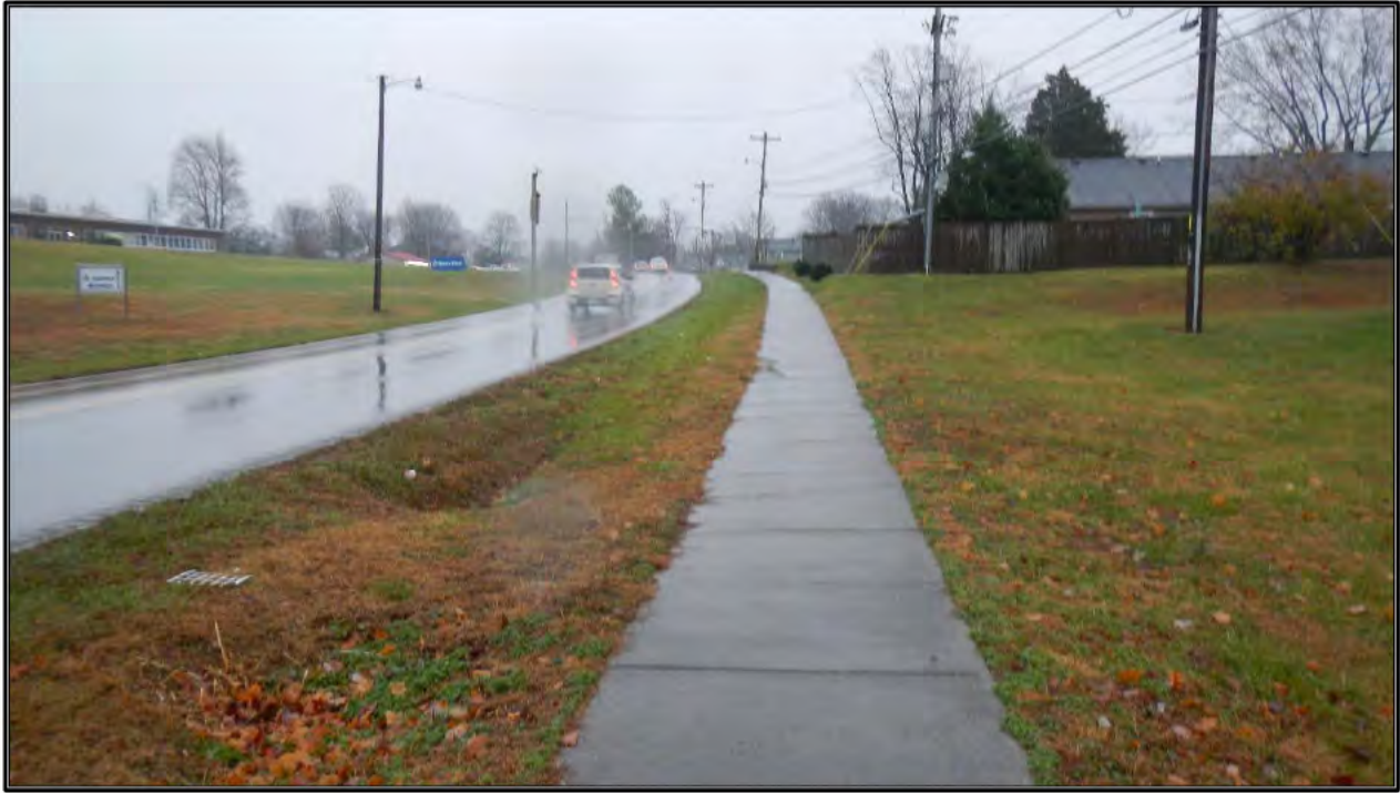
Figure 7. Sidewalk along KY 1297 (Cleveland Avenue), looking east.
